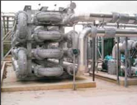
Monsal Hot Water Heat Exchanger Module
